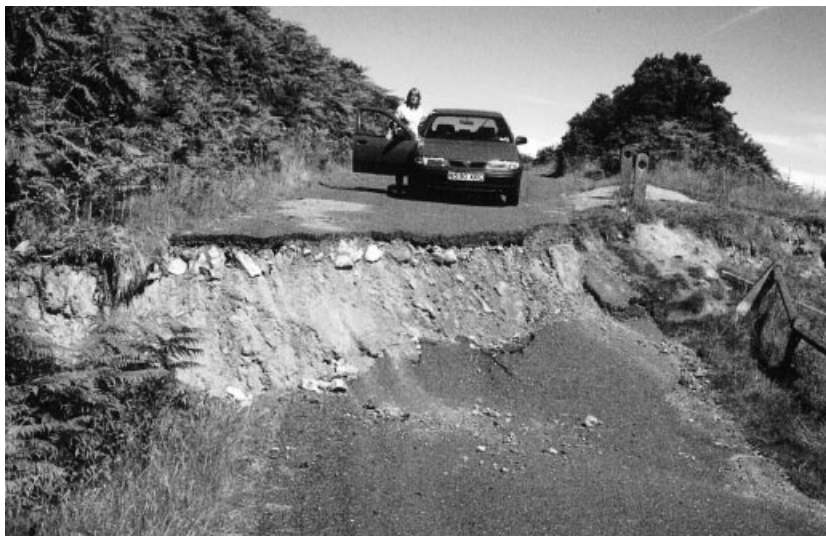
Fig. 1. Renewed movement on the landslide head scarp that has cut the road from Ainthorpe; the displacement of the road represents the downward movement of the graben across the head of the slide. (Photos by George Dowson and the authors.)
