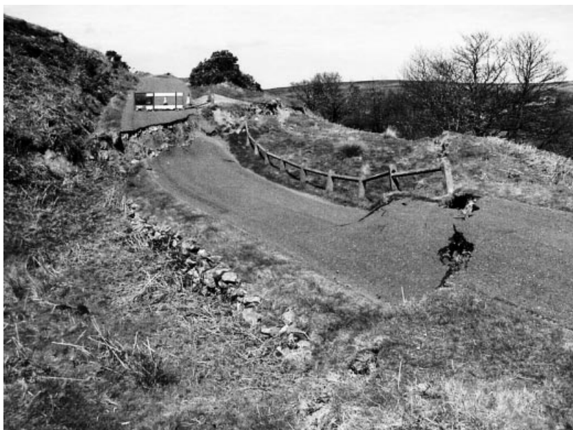
Fig. 3. (left) The graben across the road, with its higher margin on the left forming the landslide head scarp. The main slide mass on the right is moving downslope and away to the right.
