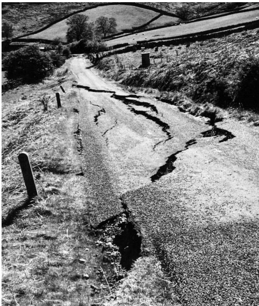
Fig. 5. Subsidiary movement within the landslide mass has created small steps in the road surface; a miniature graben has formed just below the head scarp.
